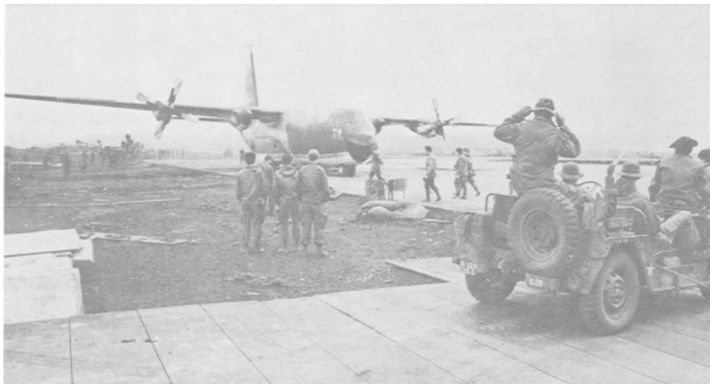
30: C-119 on newly constructed runway at Khe Sanh, February 1971
